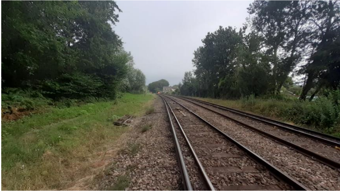
Image 1. North-facing view of the survey area. And access route from Hatches level crossing.
